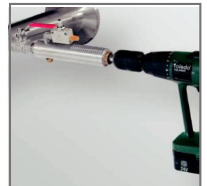
Drilling under pressure with CS drilling jig
